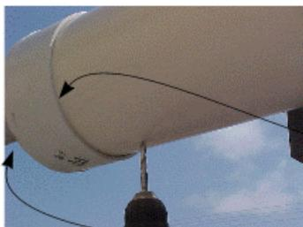
Drill drain holes in bottom of cover. Seal around tubing and
